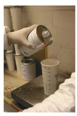
This can also be done by volume in a measuring jug or in a container with a measuring stick. It is imperative that the correct amount of hardener is put in as this affects the drying time, the adhesion, the gloss level and the elasticity and longevity of the product. Please refer to the TDS for the mixing ratio. When the paint is ready for spraying, pour it into your spray gun using an appropriate paint filter. Please note that the sparkle clear coat is not to be filtered.
